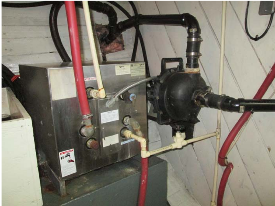
Photograph 19 - Hydraulic bilge pump and hot water heater
