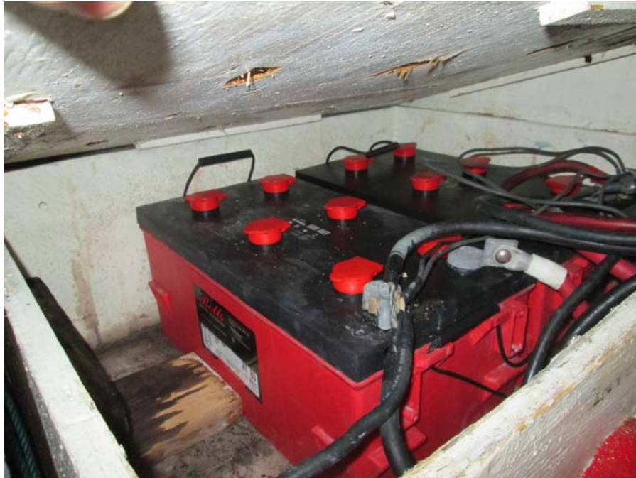
Photograph 17 - Battery bank (two of)
