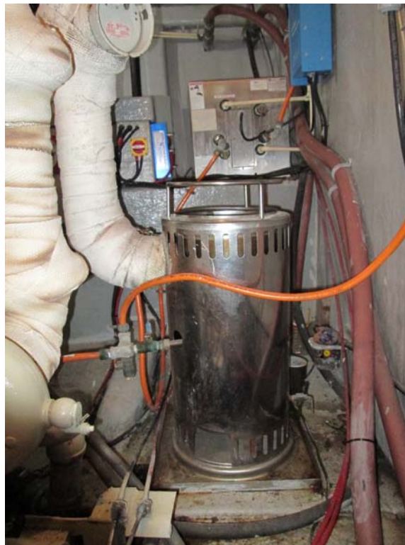
Photograph 22 - Oil / jacket water furnace
