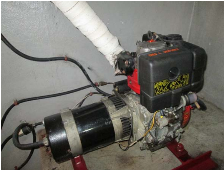
Photograph 14 - Auxiliary generator
