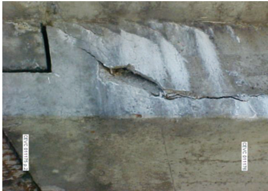
Figure 3.3 Hole and Crack in the East Abutment, photographed by Mr. Bonin between 11:45 a.m. and 12:00 p.m., September 30, 2006.
