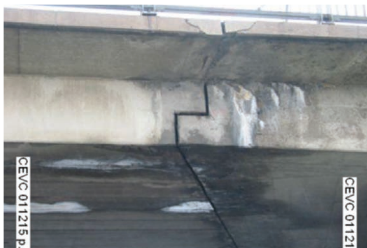
Figure 5.6 Views of the east cantilever, from the south side of the de la Concorde overpass, showing the evolution of cracks in the bearing support area 78
