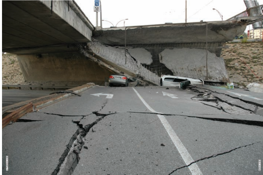
Figure 6.2 Front view of the east abutment shortly after the collapse, on September 30, 2006 2
